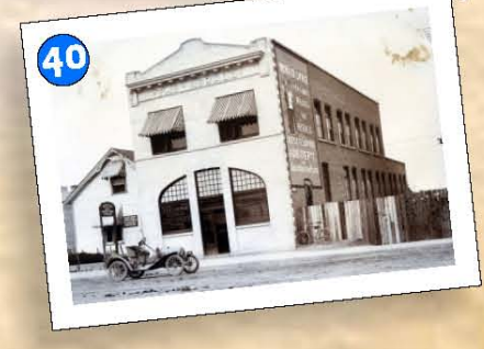
Lethbridge Herald Building 1910-1912 323 - 6 Street South. Automobile in the front and the R.C. Addison Undertaking Parlour at the side, proprietor Moore. UID 19891049200
