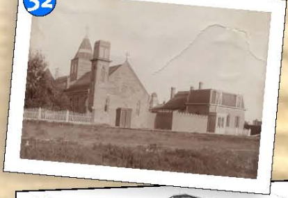
St. Patrick's Catholic Church & St. Patrick's Rectory 1898 The official opening of St. Patrick's Catholic Church was held in August 1887. It was reported by the Lethbridge News that it was the first stone church built in Southern Alberta. The church was demolished in 1950. UID 19705195003
