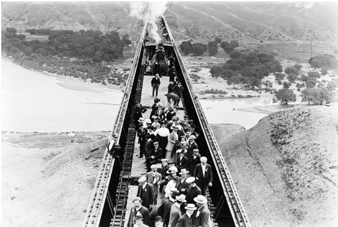
First train crossing the Canadian Pacific Railway Viaduct at Lethbridge, 1909. Galt Museum & Archives, 19640458000
