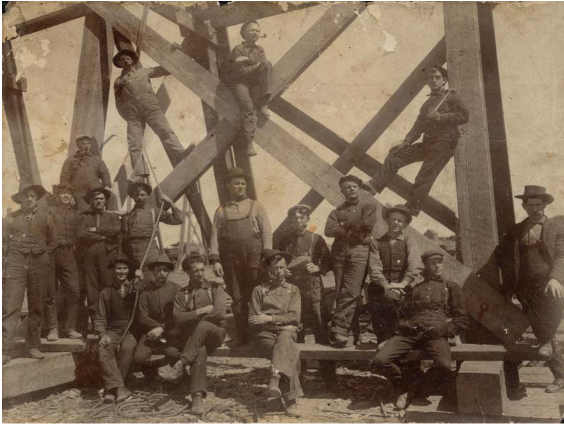
Work crew posing on the scaffold for the first span of the Canadian Pacific Railway High Level Bridge at Lethbridge, 1908. Galt Museum & Archives, 1975432000
